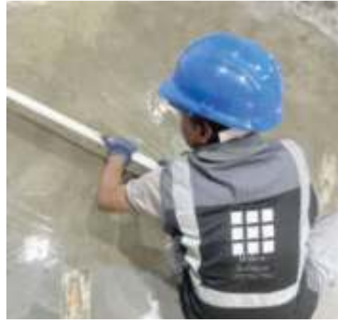
Floor Levelling / Cementing
