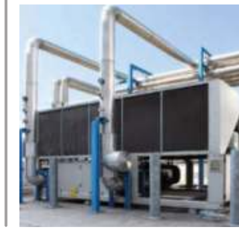
AHU's, FAHU's & VAV's
