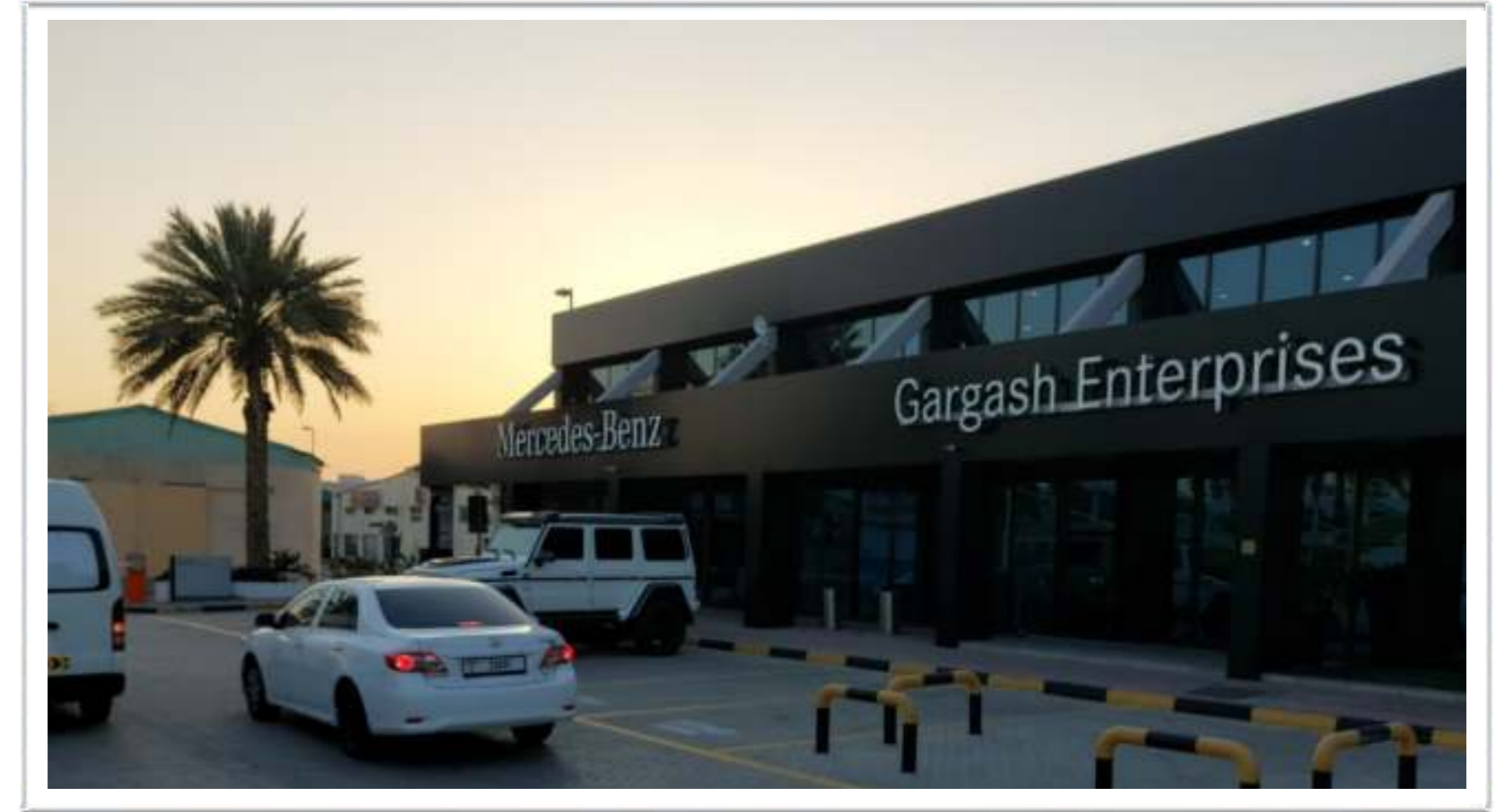
RENOVATION OF MERCEDES - BENZ CAR SHOWROOM
