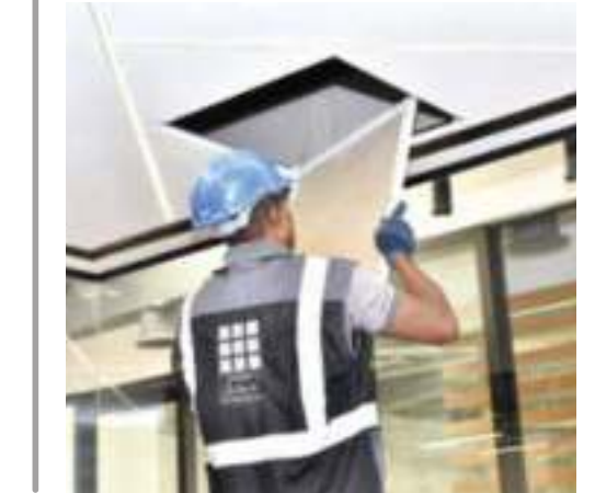
Plain Gypsum Ceiling
