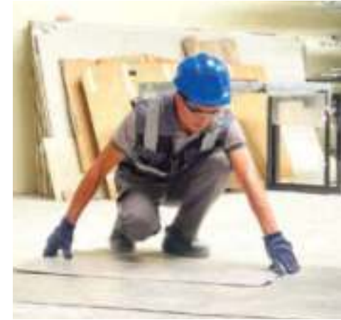
Floor and Wall Tiling
